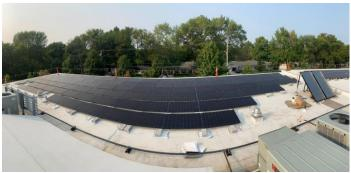
An explanation for fewer than the 270 panels originally projected is that the newer panels that were installed have more photovoltaic capacity than the assumed capacity per panel when the building was designed in 2015.
